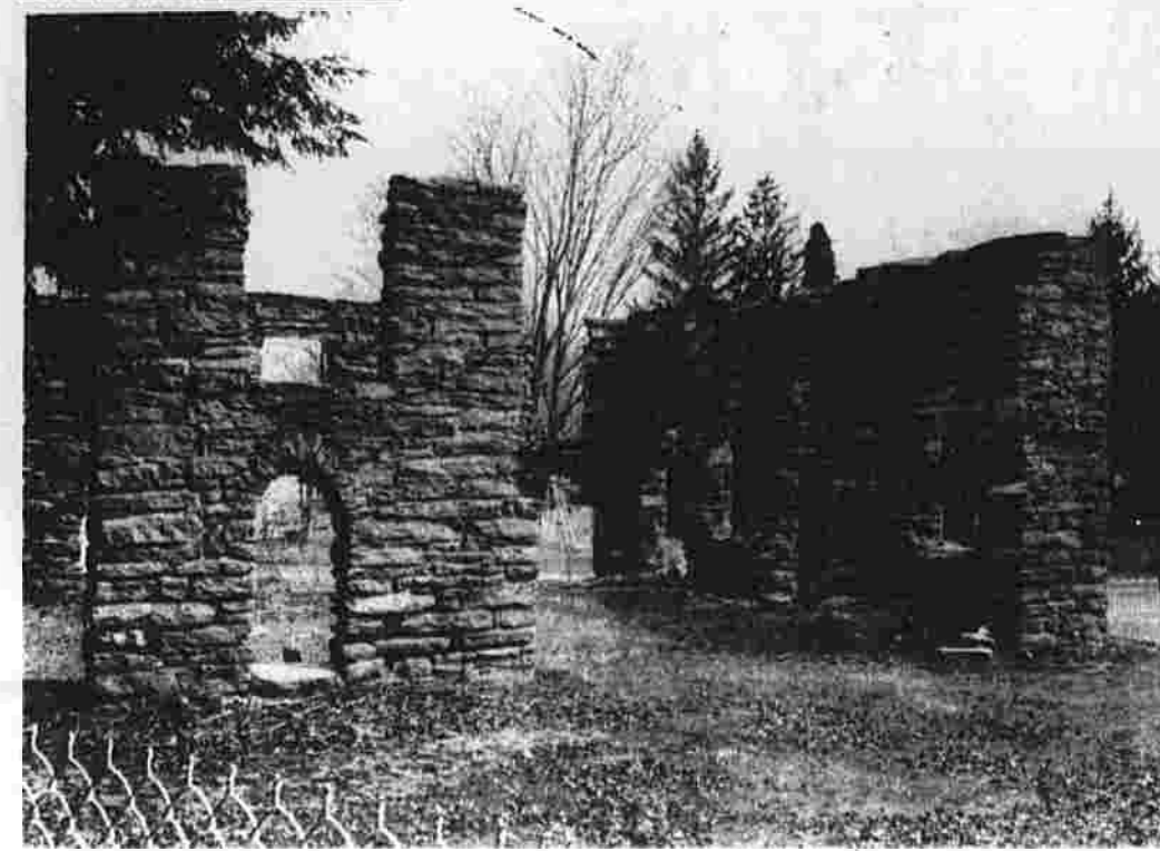
One of the first projects planned by the Pitkin Glass Works, Inc. is the pointing of the stone. In so doing, the corporation hopes to strengthen the walls so they can support reconstruction. (Herald photo by Kearns)
