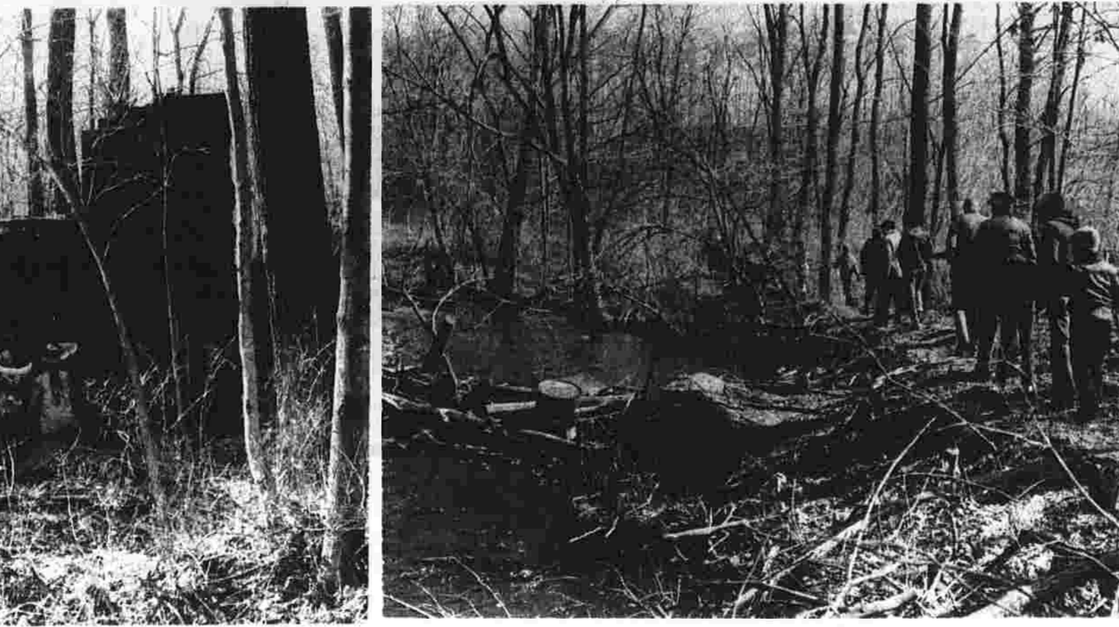
dikes and ponds which were an integral part of the mill and what contributed to the original disruption and pollution of the river.
